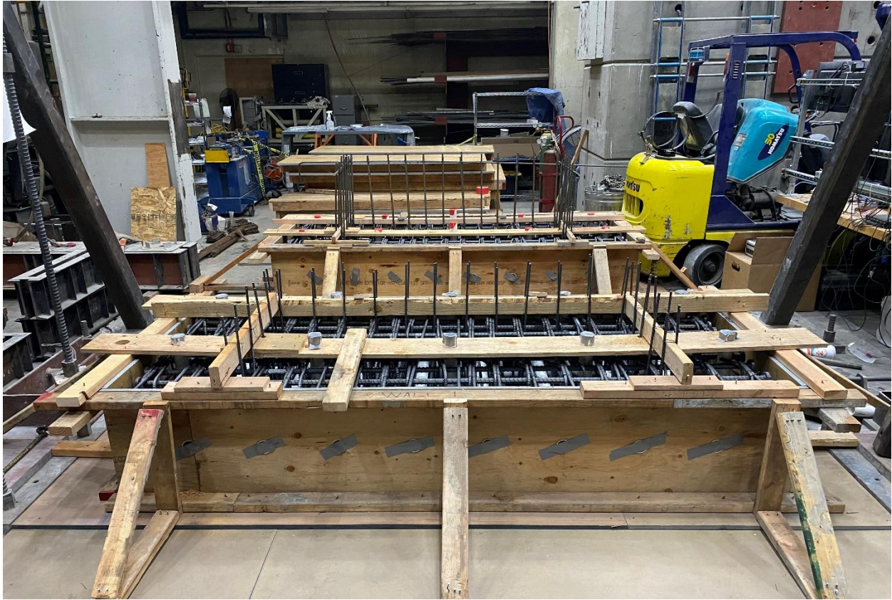
Figure D-1: Footing formwork, (Bottom) CW-1, (Top) CW-2
