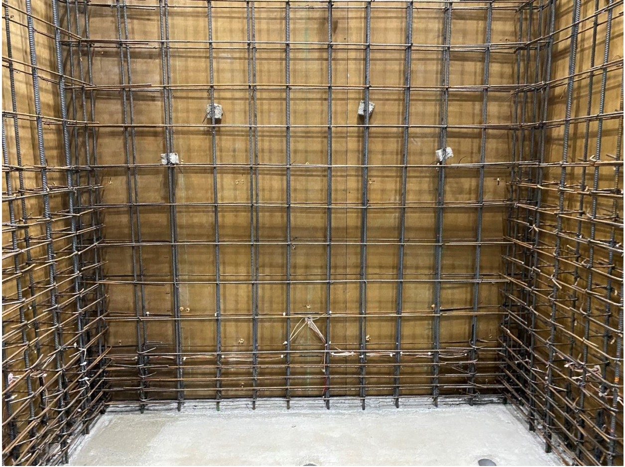
Figure D-3: CW-1 Rebar Cage
