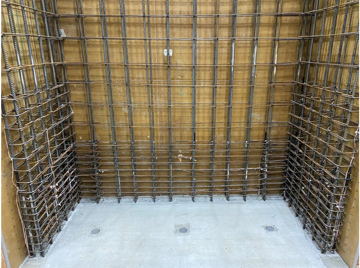
Figure D-6: CW-2 rebar cage
