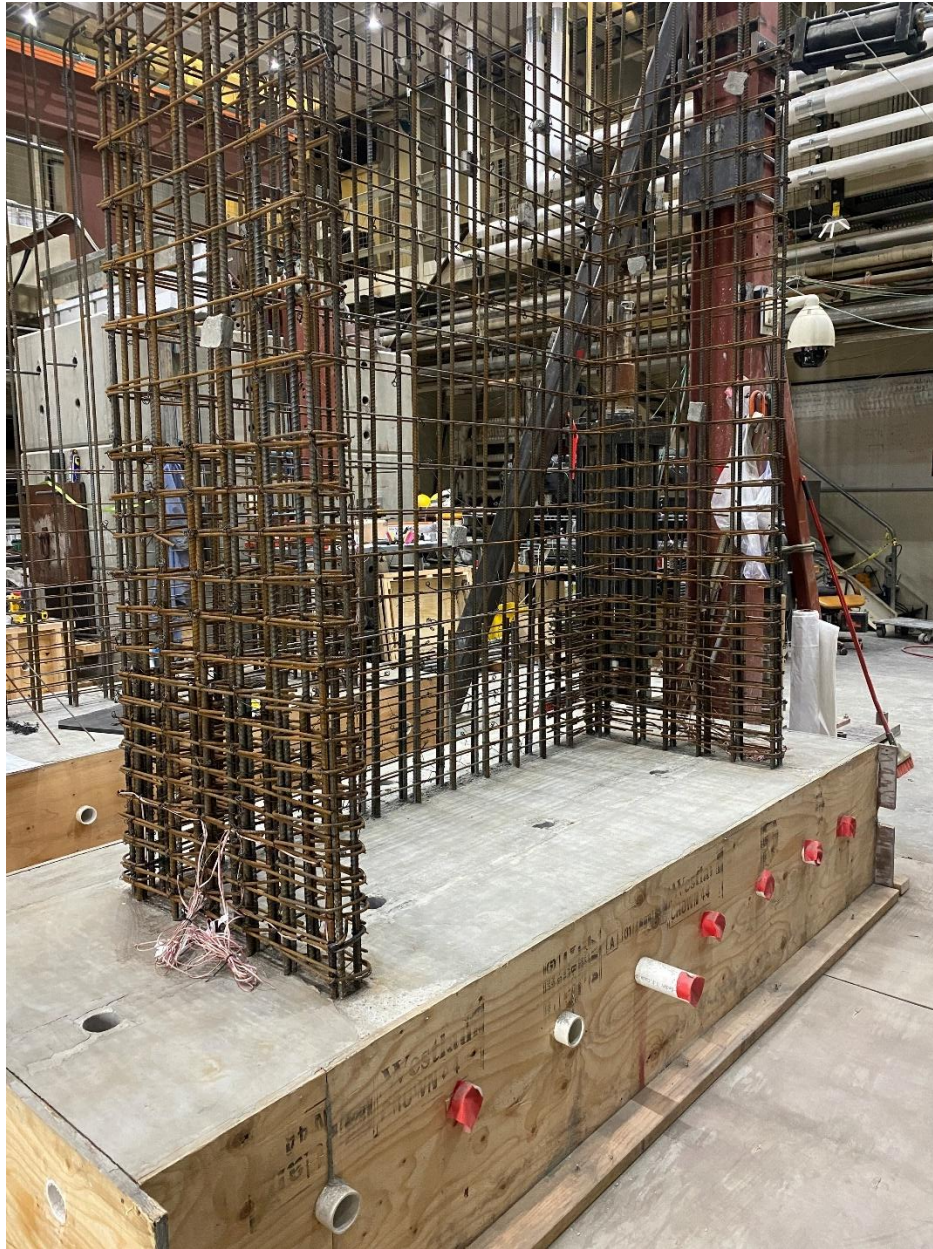
Figure D-10: CW-3 Reinforcement cage
