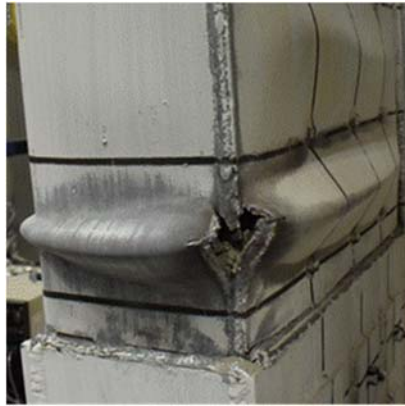
Figure 4-21. Vertical weld fracture at the corner of the NWS and NWW surfaces
