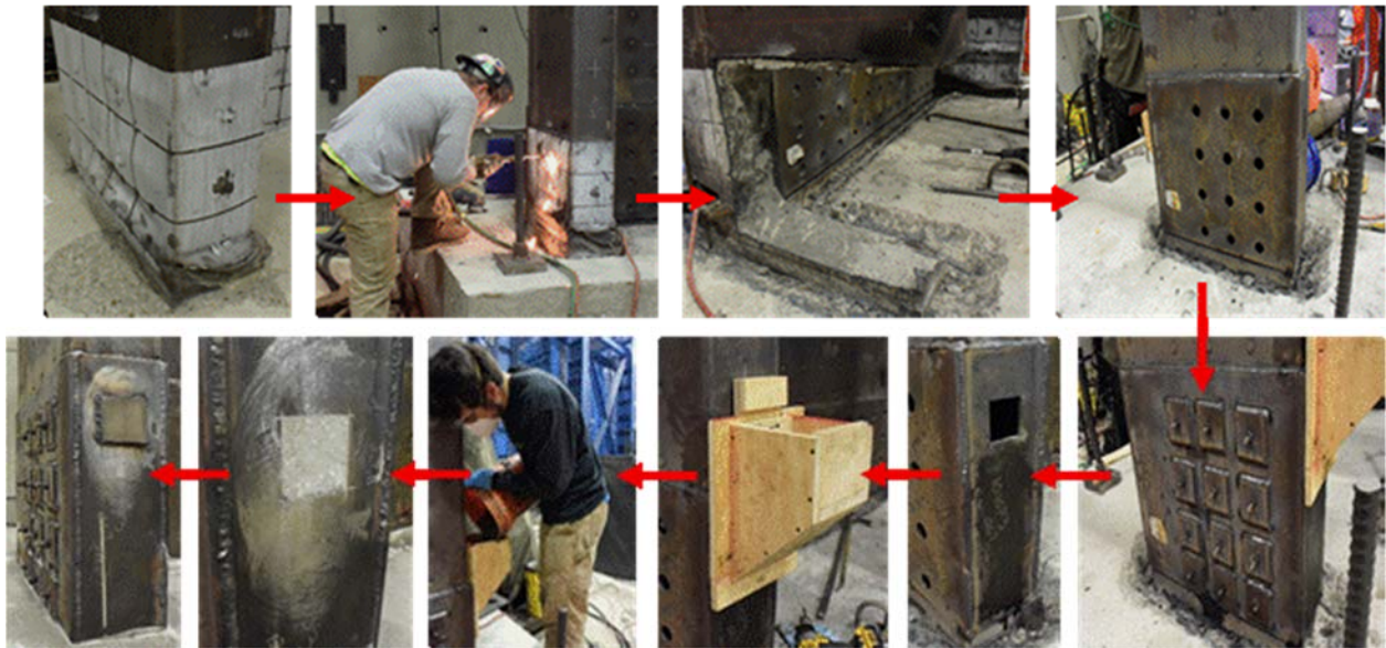
Figure 4-6. Repair sequence of webs
