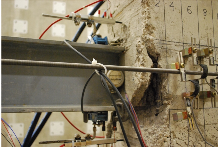
Figure 3.3 State of connection at the conclusion of testing – specimen 1a (test 1).
