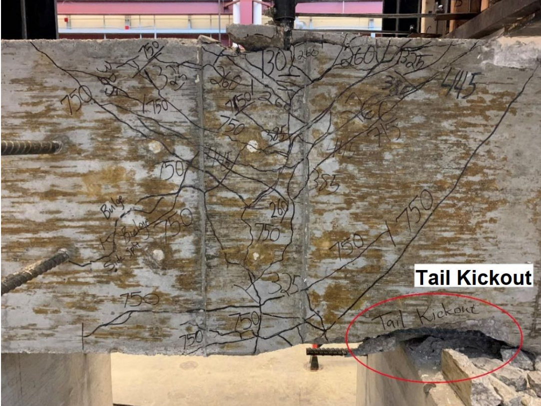
Figure 3.5 Side view of a concrete breakout failure in hooked bars with tail kickout (H14-7)
