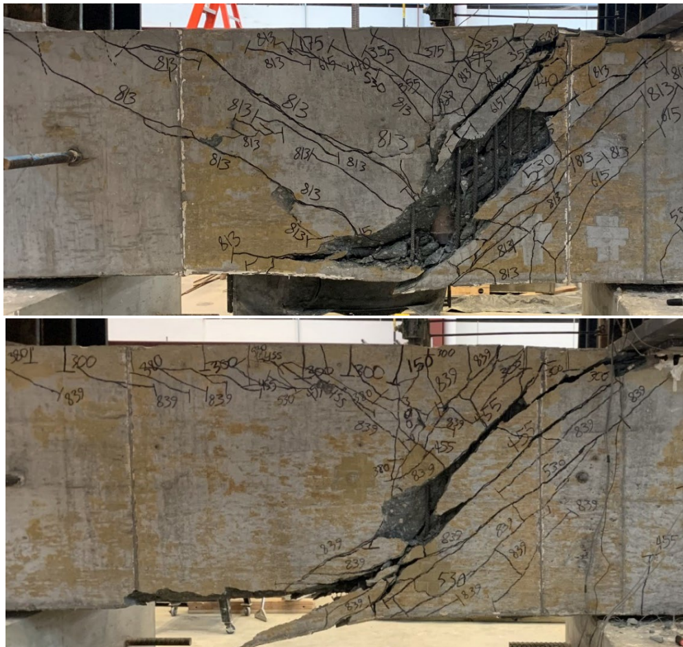
Figure 5.31 Comparing failure modes of specimen 18-2 with 3.5 in. side cover to the bar (top) with specimen 18-6 with 6.5 in. side cover to the bar (bottom), both with A_{tl}/A_{hs} = 0.543
