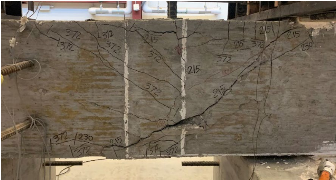
Figure 5.15 Anchorage failure observed in specimen 14-15 ( A_{tr}/A_{hs} = 0 ) tested under loading condition B
