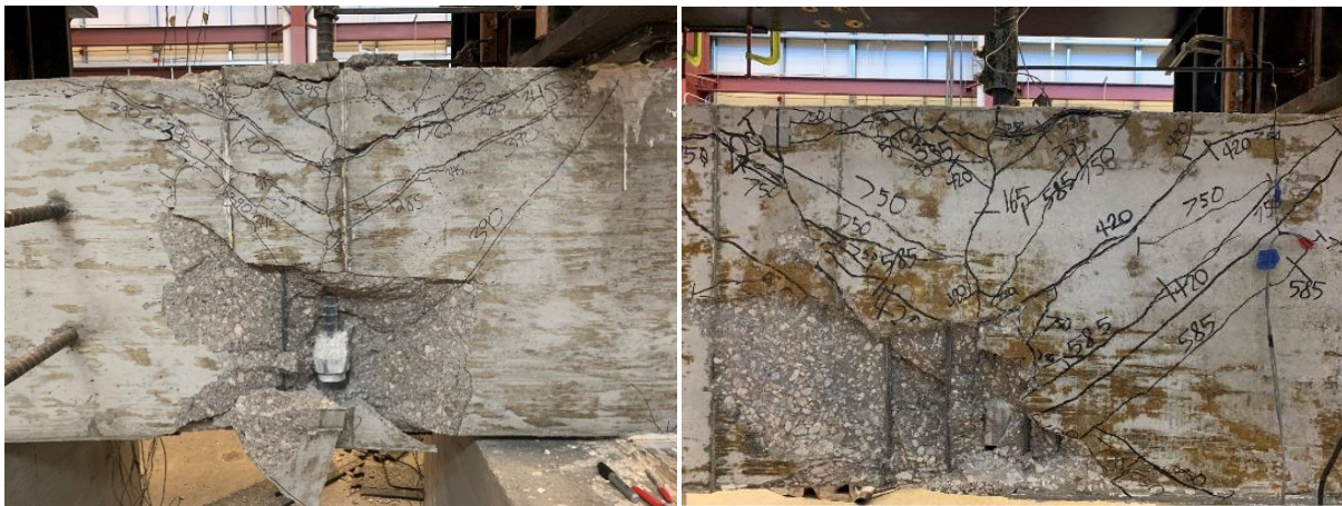
Figure 3.8 Primarily side-splitting failure (left: specimen 14-3, right: specimen 18-4)
