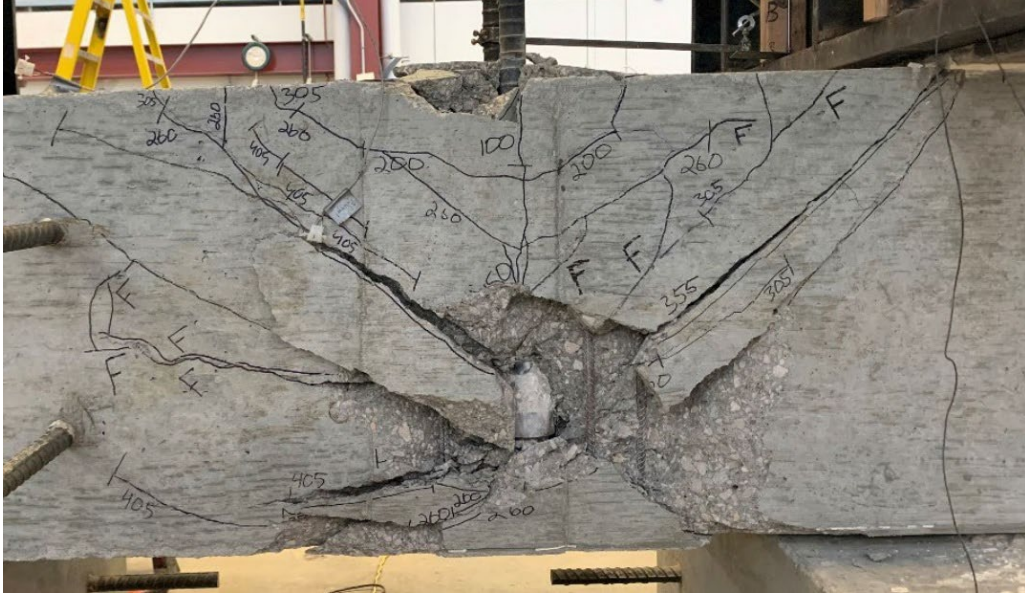
Figure 5.21 Anchorage failure observed in specimen 14-16C ( A_{tr}/A_{hs} = 0.356 ) tested under loading condition B
