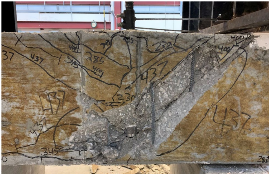
Figure 5.24 Anchorage failure observed in specimen 14-16E ( A_{tt}/A_{hs} = 0.551 )
