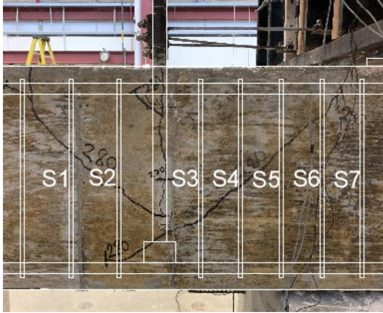
Figure 3.14 Parallel ties trapping the first diagonal cracks and their strain gauge labels in the headed bar specimen 14-6
