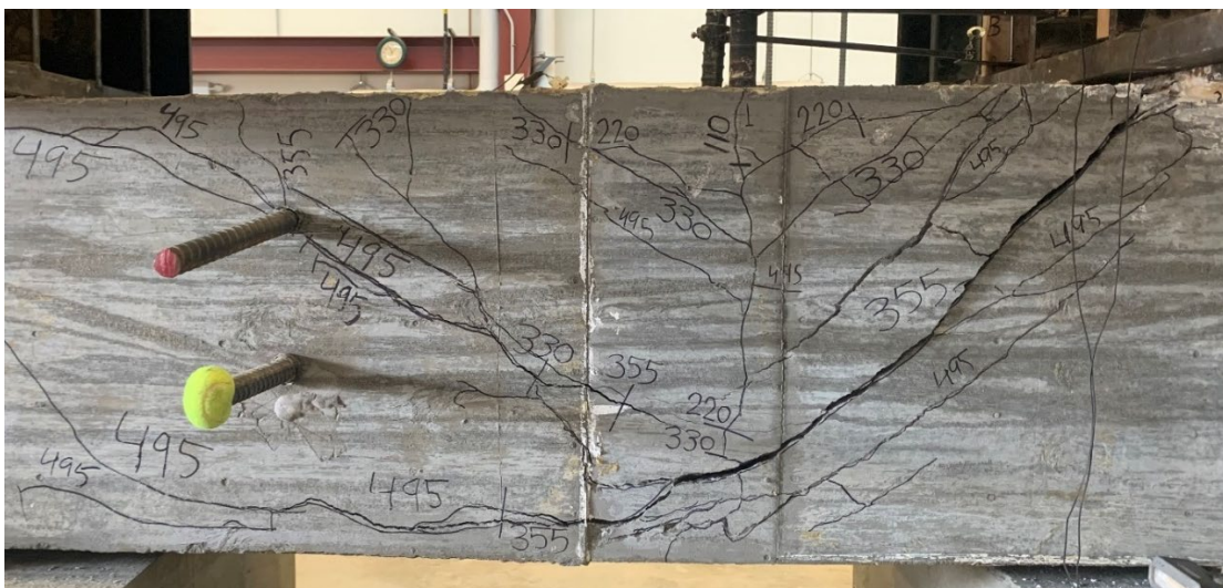
Figure 5.19 Anchorage failure observed in specimen 14-2A ( A_{tt}/A_{hs} = 0.267 ) tested under loading condition B
