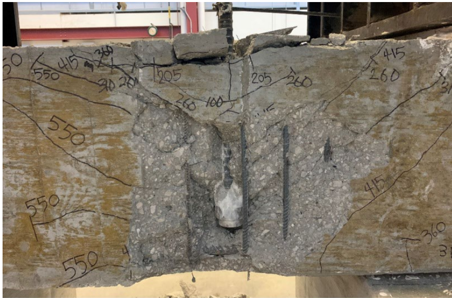
Figure 5.23 Anchorage failure observed in specimen 14-16D ( A_{tl}/A_{hs} = 0.827 ) tested under loading condition A (after removal of loose concrete)
