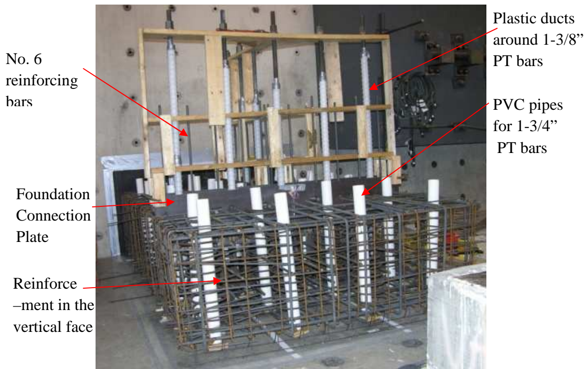
Figure 6.16 Foundation reinforcing bar cage before enclosed by forms
