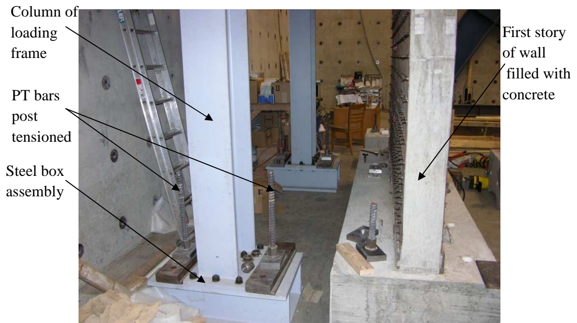
Figure 3.27 Anchoring the loading frame to the strong floor
