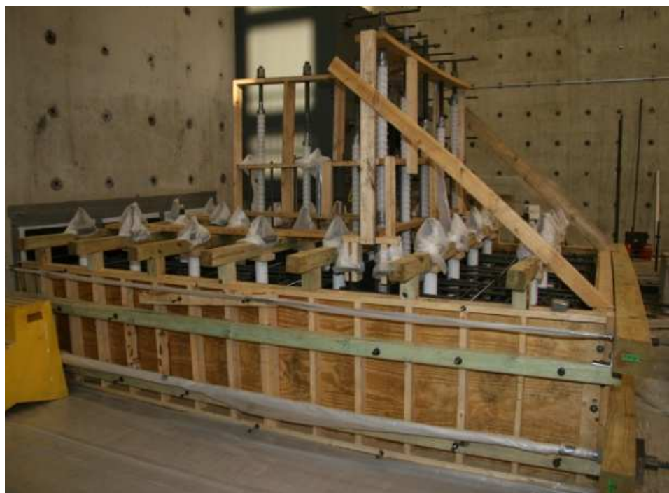
Figure 6.21 Foundation formwork before casting concrete
