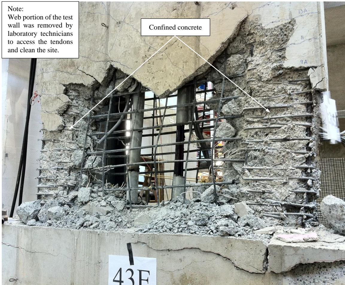
Figure 4-37 Confined concrete on the flange sections of Wall 1
