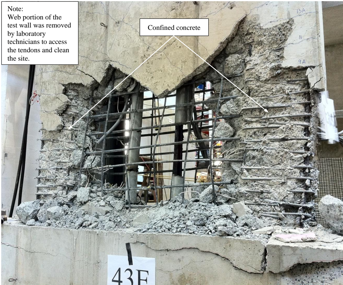
Figure 5-35 Confined concrete in the flange portions (boundary element) of the wall
