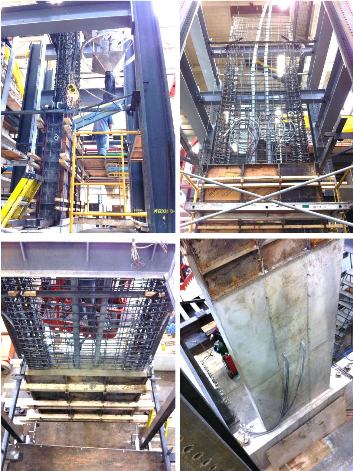
Figure 3-24 Additional construction photographs
