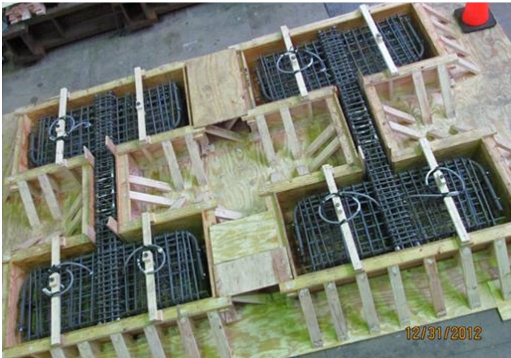
Figure 3-45: Reinforcement of testing specimens placed inside the wooden forms
