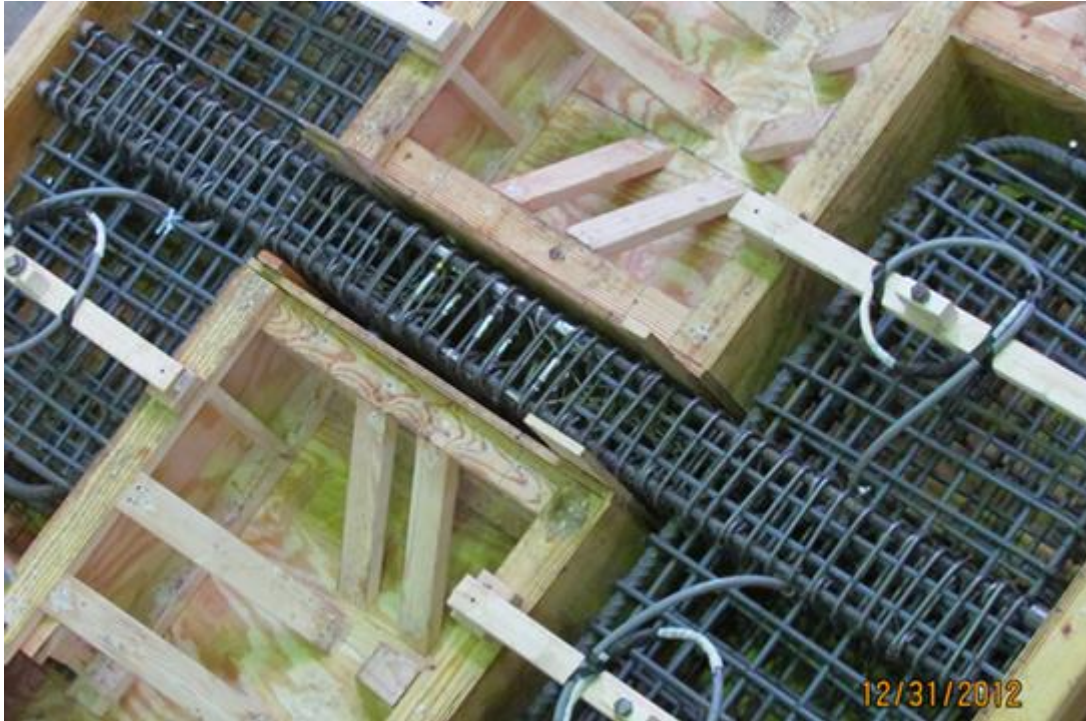
Figure 3-44: Reinforcement of confined concrete column inside the wooden form
