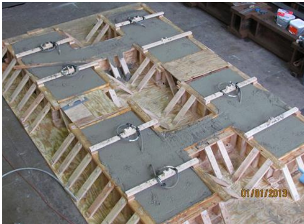
Figure 3-47: Concrete casting of test specimens
