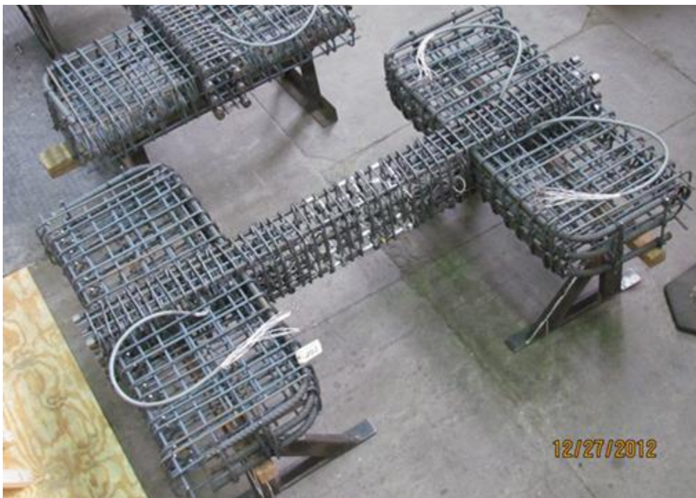
Figure 3-36: Reinforcement of TS02
