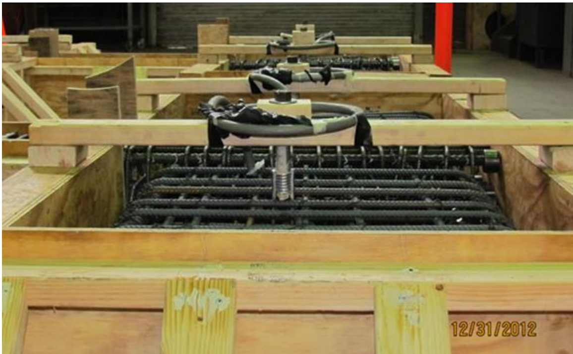
Figure 3-42: Lifting inserts installation
