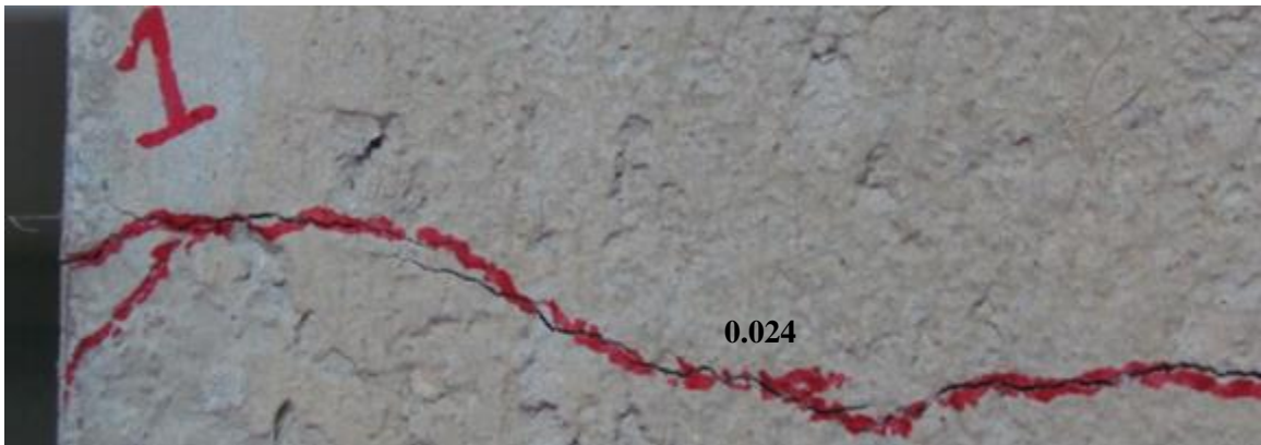
Figure 4-98: Cracks on west face of TS02 at Load Step 21
