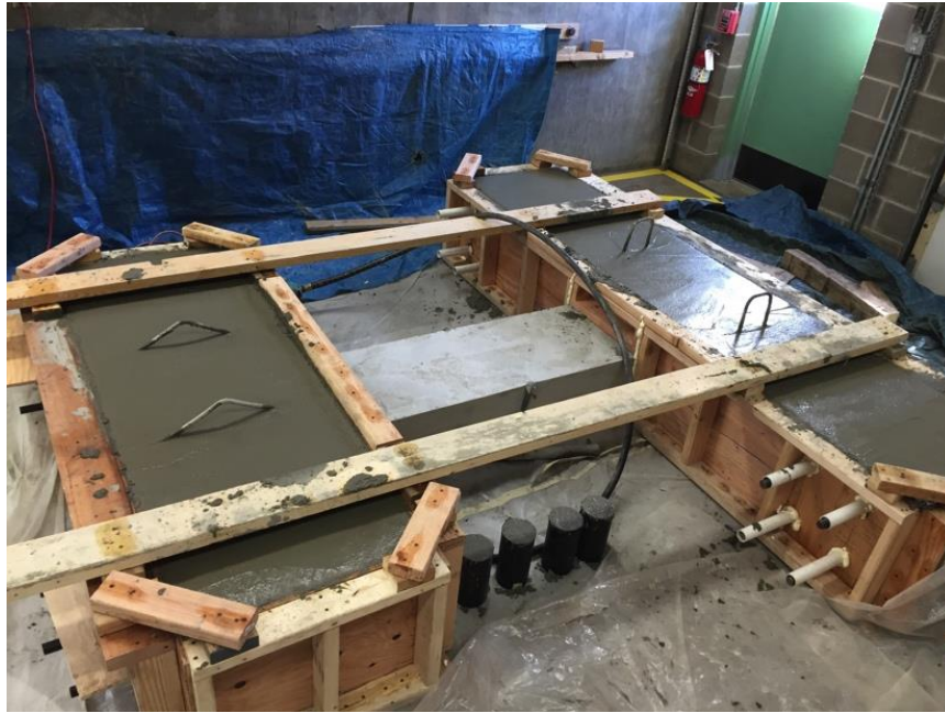
Figure 2.11: Finished Coupling Beam Specimen
