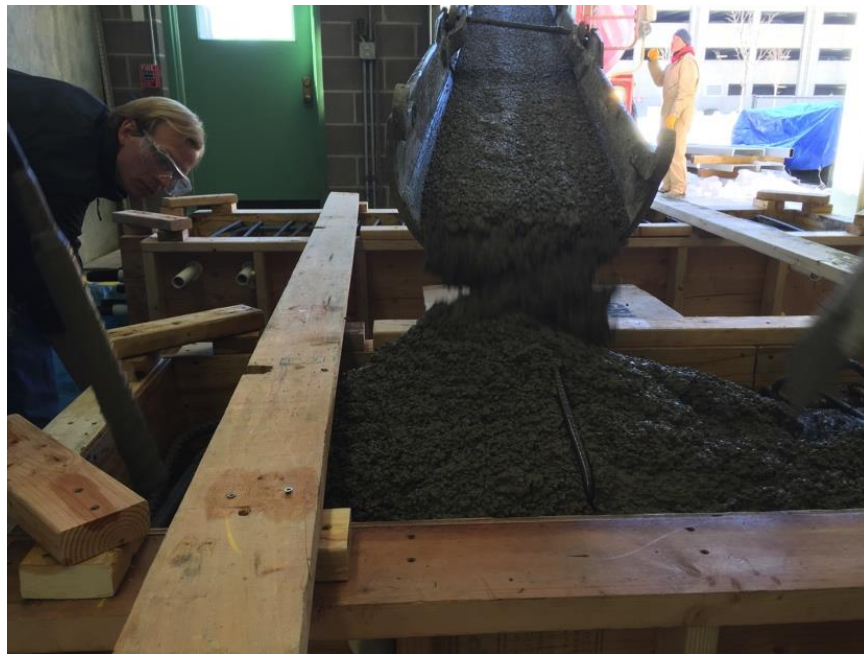
Figure 2.10: End Blocks Being Cast
