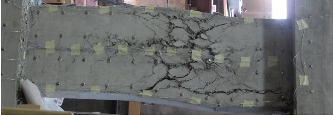
Figure 4.1: Shear Failure of Specimen CB1
