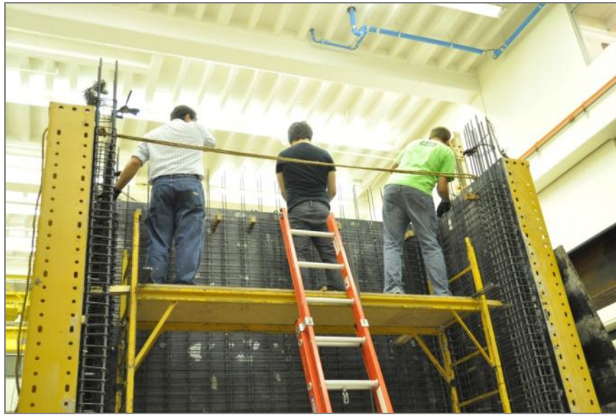
Figure 2.6: Near completion of Wall 8 rebar cage
