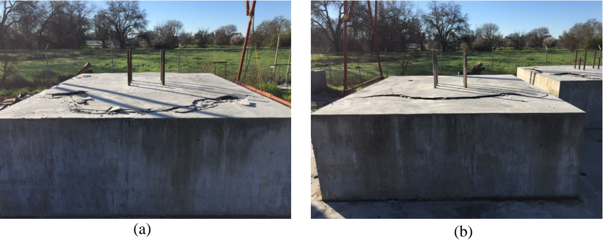
Figure 6 – Profile view of breakout surface for (a) 12-inch embedment and (b) 18-inch embedment
