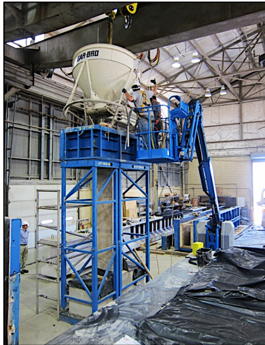
Figure 10: Column casting process
