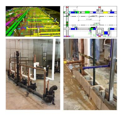
Figure 8 Example of prefabrication of piping systems deeply integrated with a CMU wall. Clash detection used for identification of safe regions for penetration sleeves. Images courtesy of Scott Conwell and the International Masonry Institute (http://www.imiweb.org).
