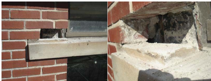
Figure 9-26. Exploratory opening.
