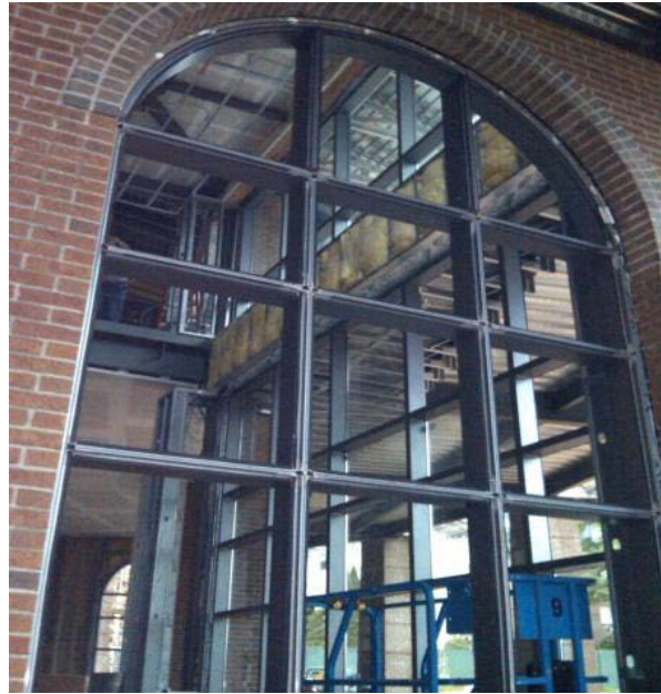
Figure 10-8. Masonry arch window.
