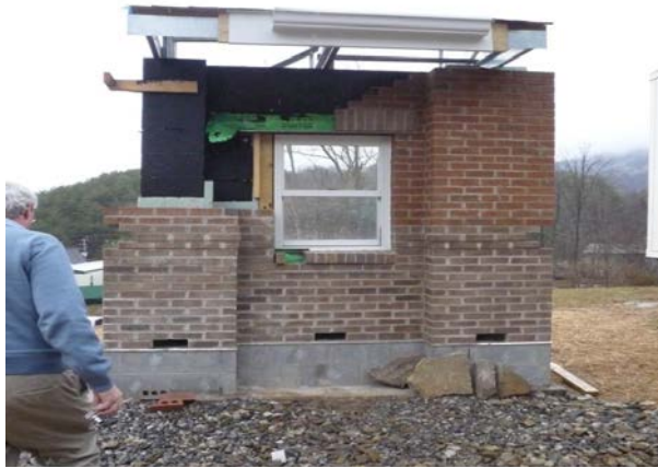
Figure 10-3. Mockup of masonry wall system.
