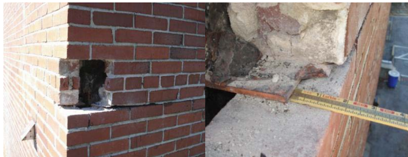
Figure 9-27. Exploratory opening.
