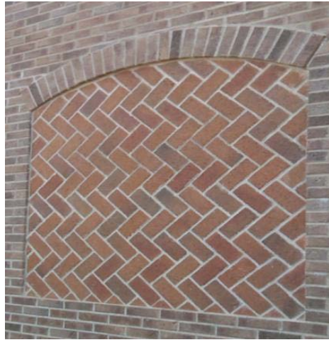
Figure 10-6. Segmental arch with herringbone pattern.
