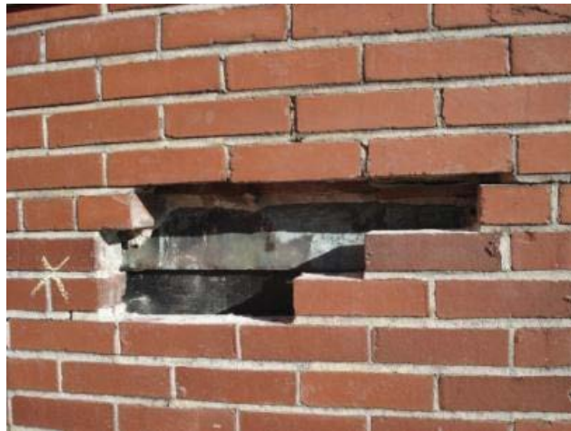
Figure 9-24. Exploratory opening.
