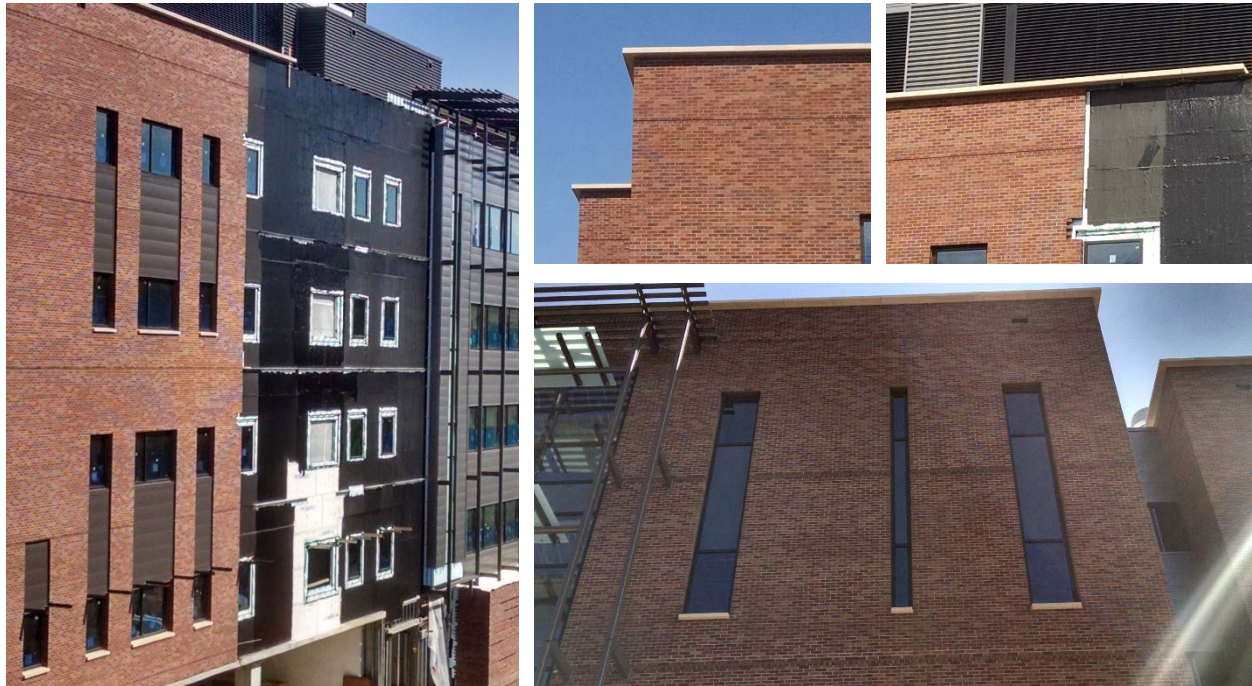
Figure 4-1. Cast stone elements on the EBB.
