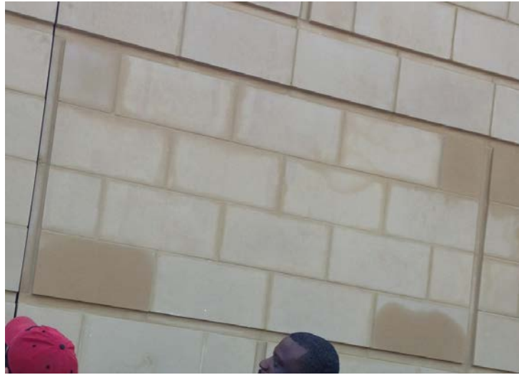
Figure 6-15. Cast stone block modification.
