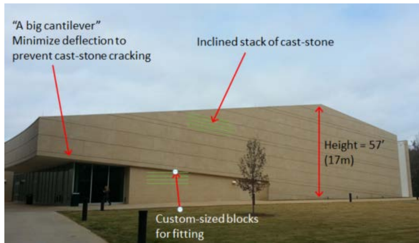
Figure 6-16. Cast stone features.
