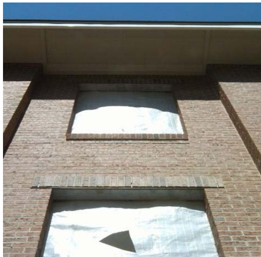
Figure 10-7. Flat gauge arch.
