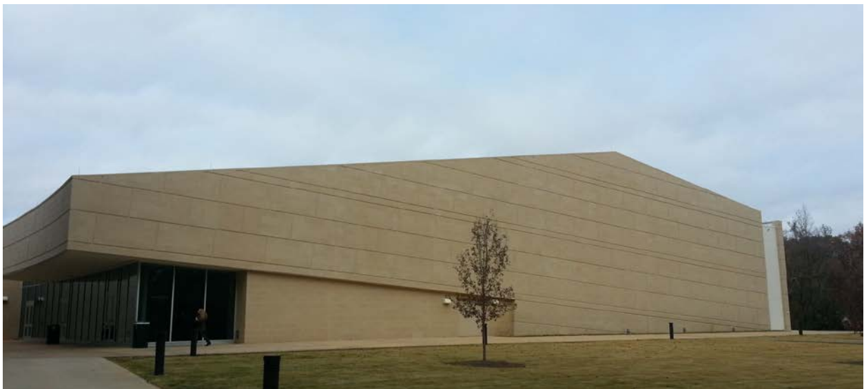
Figure 6-14. Cast stone installation on auditorium.
