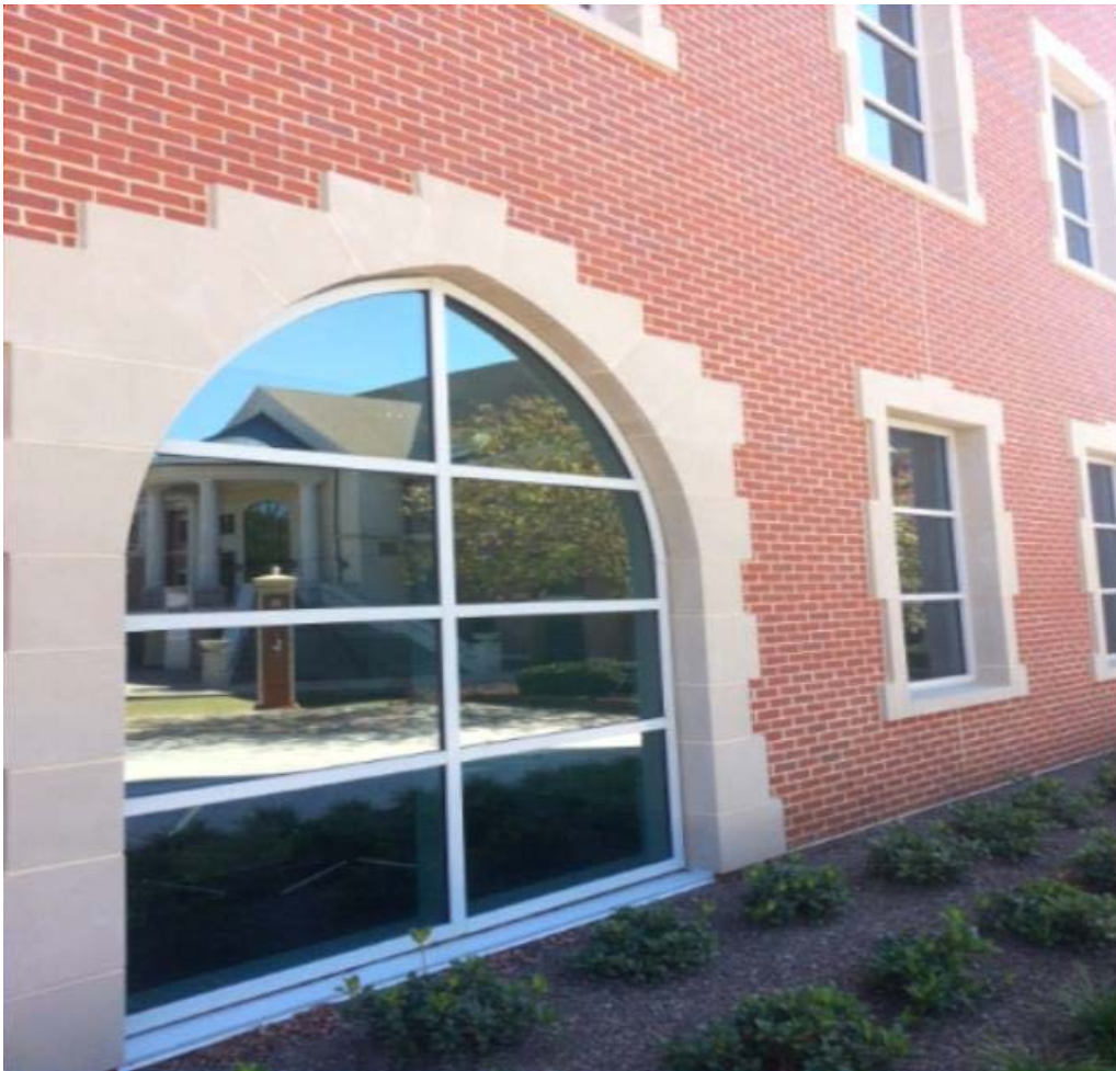
Figure 7-2. Masonry structures on campus.
