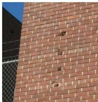
Figure 9-8. Abandoned anchor holes in east elevation of High Bay.
