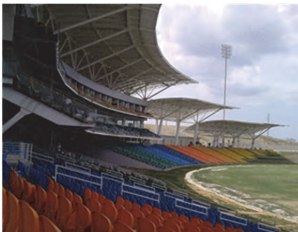
Figure 1-2 Final built construction.
