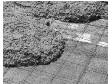
Pouring a concrete topping on a precast slab
